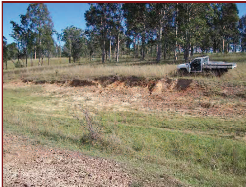
Photo 14 – Localised minor erosion in the central portion of the site
